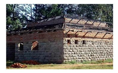
Notice the exceptional building materials using stone and bricks for a building that will endure through the ages. As the work continues, the next phase will be to install doors, windows, and a smooth plaster for the interior walls.
